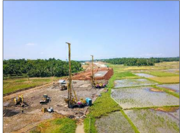
Fig. 5. Keller Installing Stone Column in Paddy Field.
