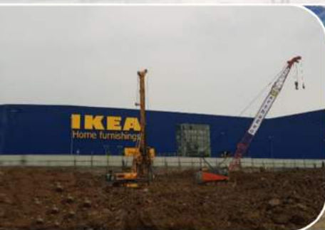
Skyhouse Bored Pile, 2019
