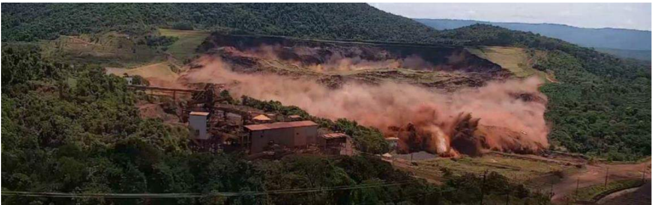
Fig. 6. Failure of the Feijao Tailings Dam due to Static Liquefaction in 2019, Robertson et al. (2019).
