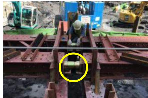
Fig. 2. Load Cell Installation.
