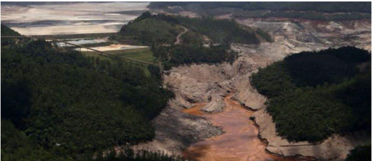
Fig. 7. Failure of the Fundao Tailings Dam due to Static Liquefaction in 2015, Morgenstern et al. (2016).
