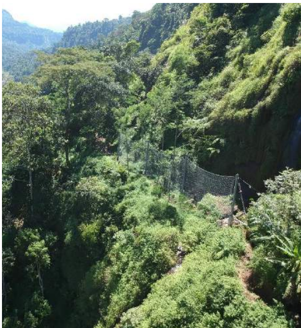
Fig. 8. The Installed Rockfall Barrier Protecting the Infrastructure Below.
